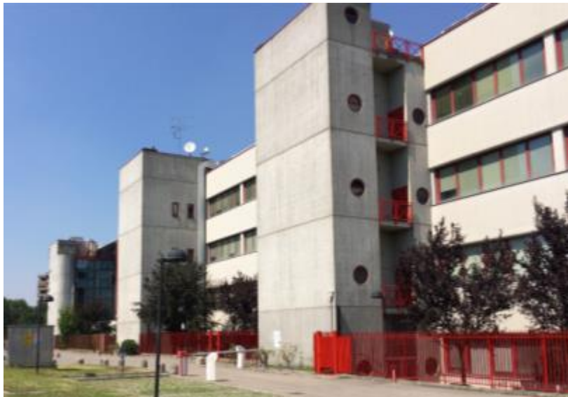
Master-leased facilities such as Milan Data Centre (in picture) enhance the REIT's income stability and visibility
