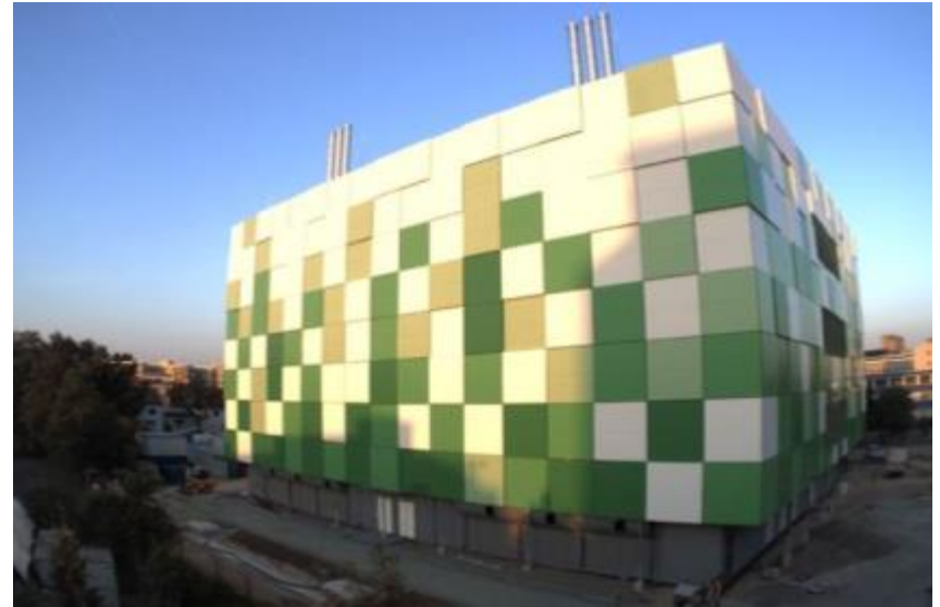
maincubes Data Centre on track in Germany
