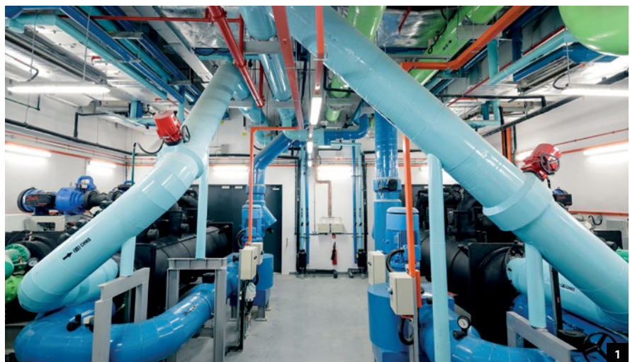
1. The report scope outlines practices in Keppel DC REIT's colocation data centre assets that the Manager has operational oversight of.
