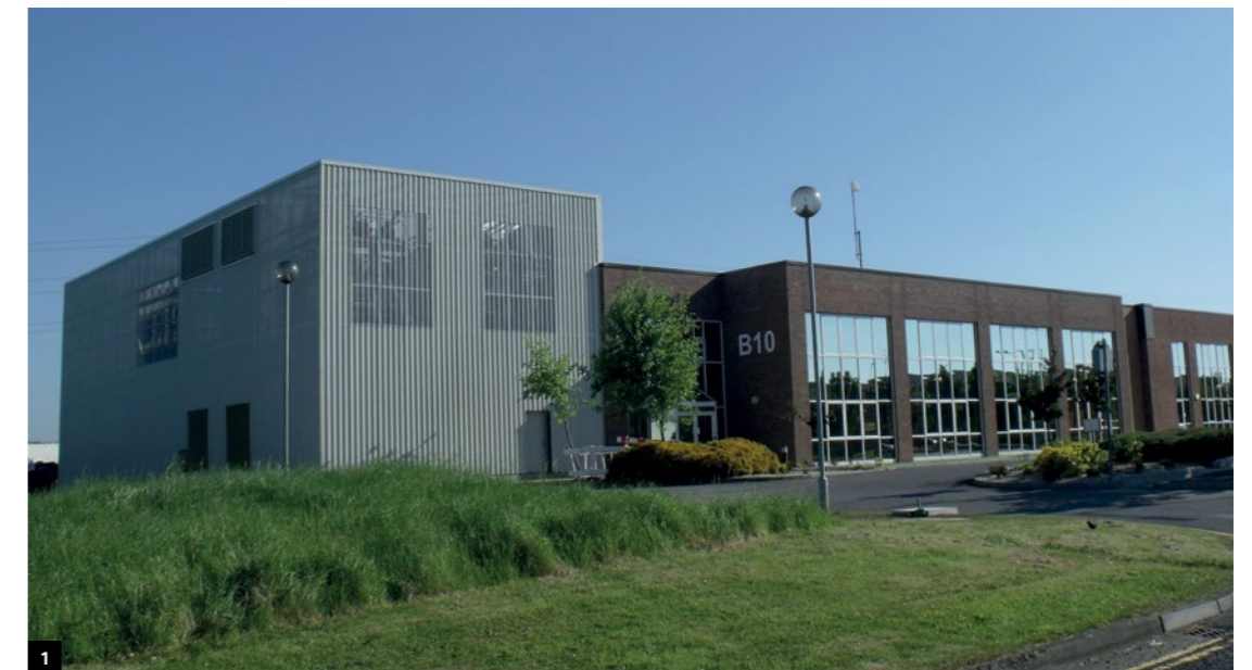
1. The REIT acquired its second data centre asset in Dublin, Keppel DC Dublin 2 (formerly B10 Data Centre).
