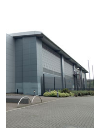
Cardiff Data Centre
