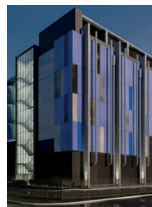
Intellicentre 3 East Data Centre (Under development)
