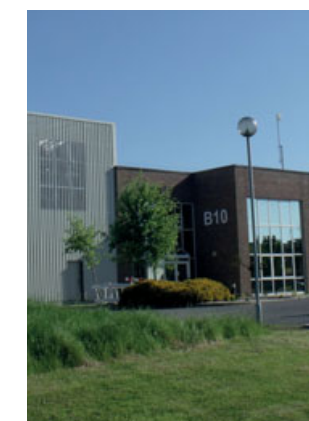
Keppel DC Dublin 2
