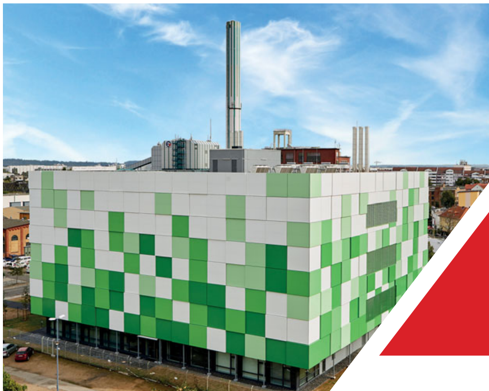
maincubes Data Centre is 10km from Frankfurt, one of the leading European data centre markets.
