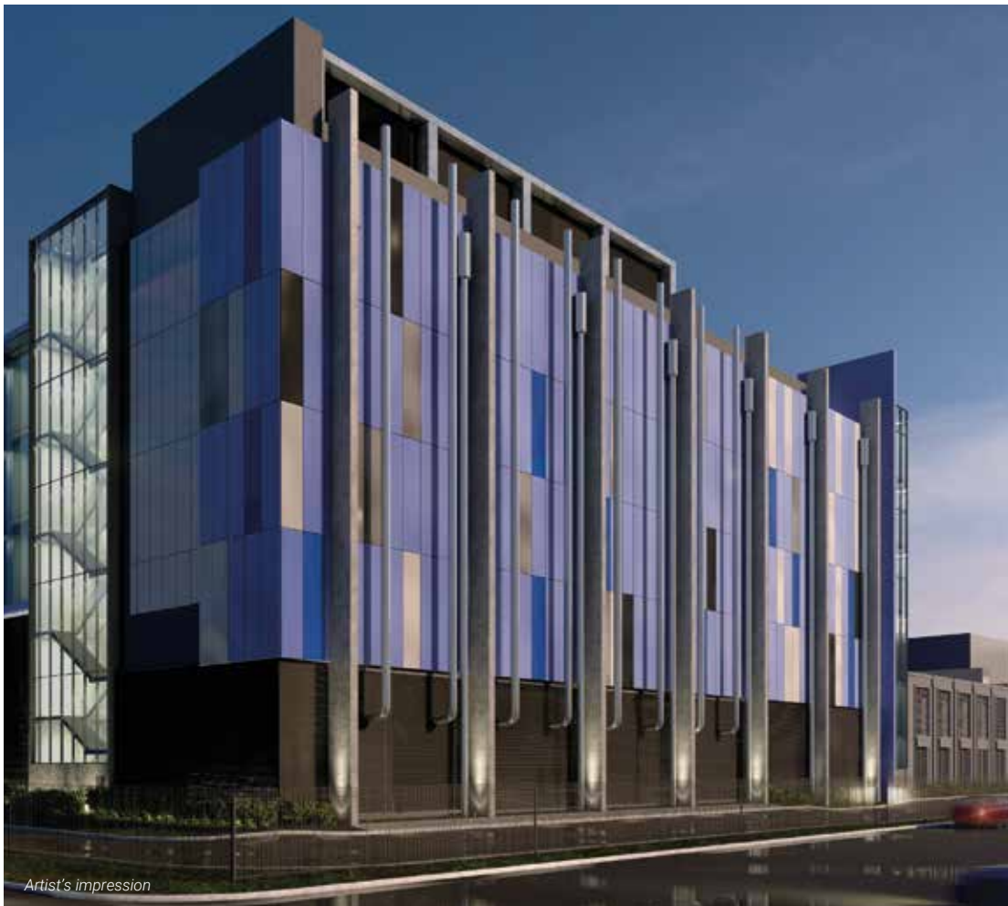
Intellicentre 3 East Data Centre will be built on the vacant land within Intellicentre 2 Data Centre's site.
