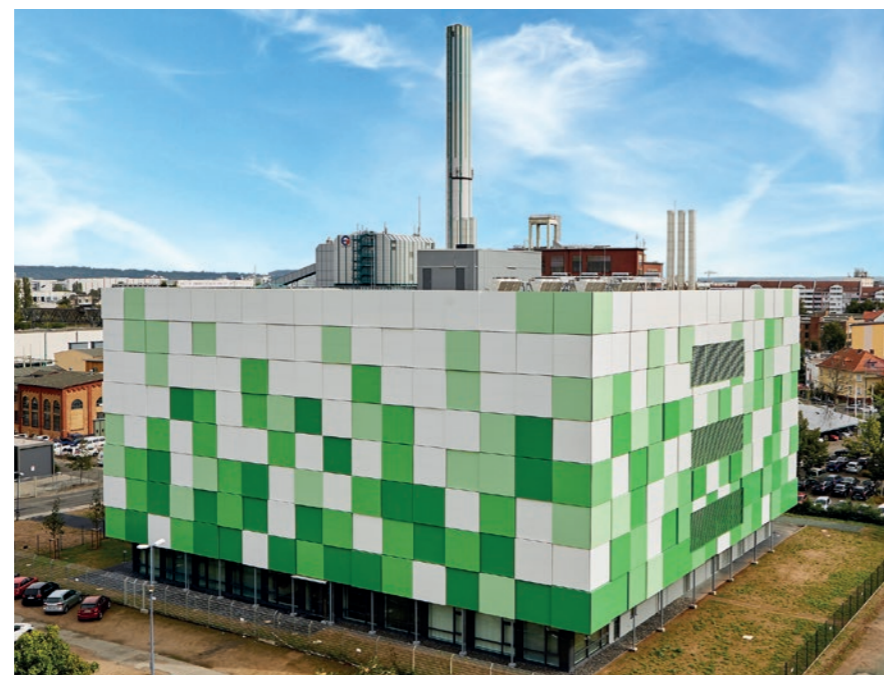
Keppel DC REIT completed the acquisition of maincubes Data Centre in Offenbach am Main, Germany, in March 2018.
