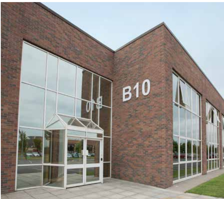
Keppel DC Dublin 1 and Keppel DC Dublin 2 continue to be fully powered by wind energy.
